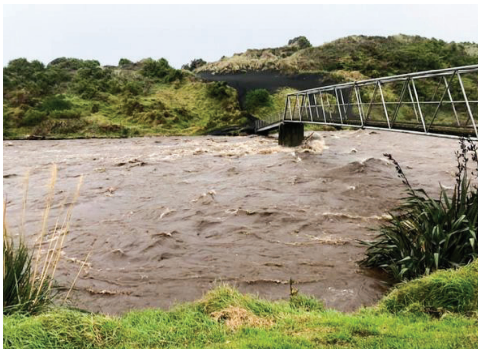
Kaupokonui River Bridge in flood.
